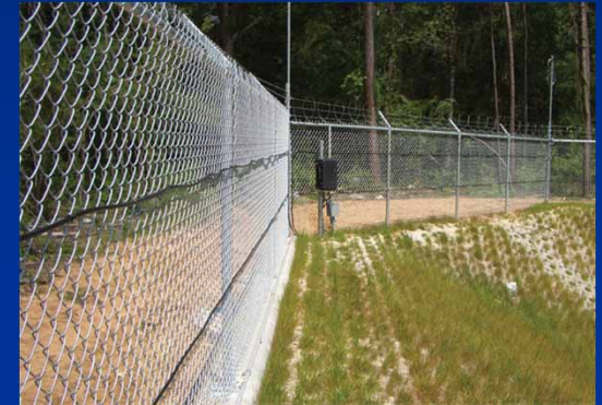
Border Security Monitoring
